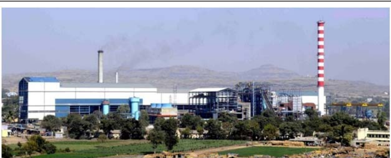
30 MW Cogen Power Plant at Sahakarmaharshi Bhausaheb Thorat Sahakari Sakhar Karkhana Ltd., Sangamner, Maharashtra.
